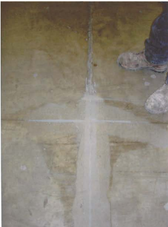
RAZOR OFF CURED SPAL-PRO 2000 OVERFILL
