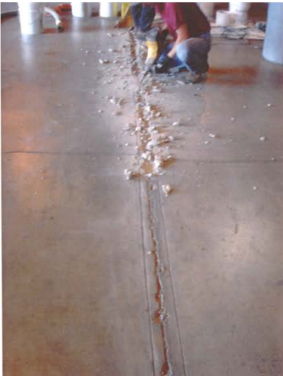
REMOVE REMAINING CONCRETE
