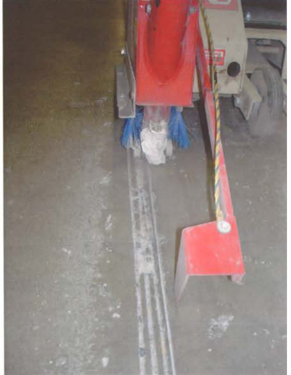
PRIME CLEANED JOINT WITH AH LIQUID
