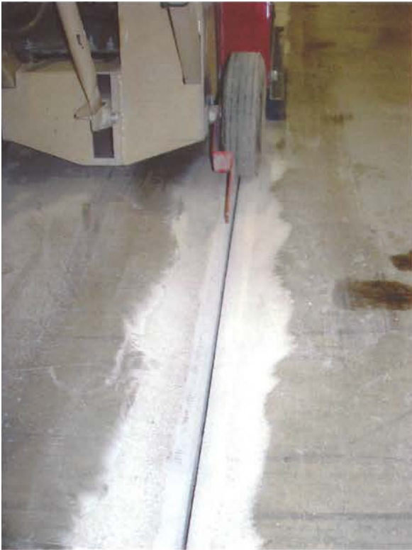
RAZOR OFF CURED SPAL-PRO 2000 OVERFILL
