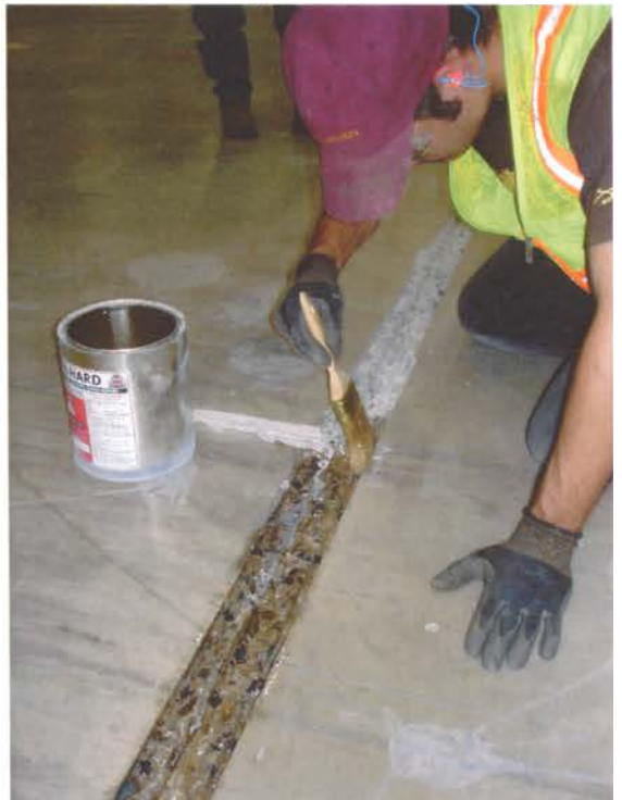
PRIME CLEANED JOINT WITH AH LIQUID
